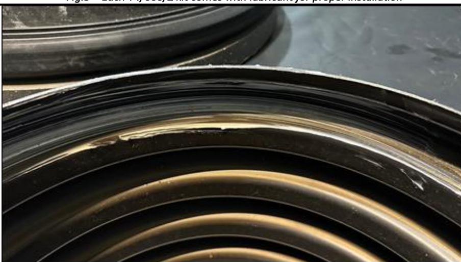
Fig.4 – Implementation of lubricant to facilitate gasket installation in the internal cavity of the corrugated pipe.
