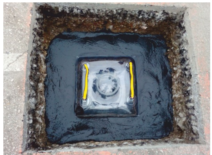
500x500 pneumatic formwork installed in a well with square cross-section.
