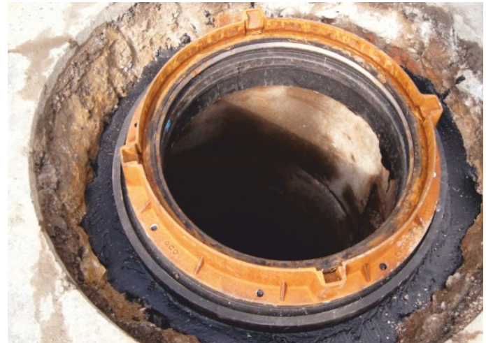
① Surface finial of DN600 sewage well with height of 24 cm consisting of mutually compatible T1R/625 and T1/600 compensation rings and T1K/600/9/22 wedge rings.
