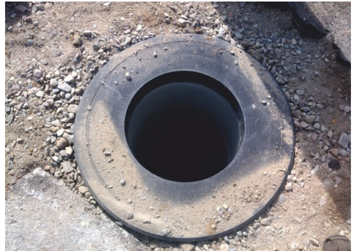
TX/765/410 adapter prepared for the assembly of a 400x600 street drain, placed on a DN450 concrete rain water well.
