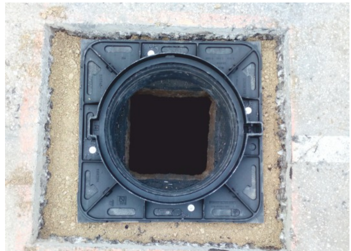
Ductile cast iron manhole with square body plate of 850x850mm set on a T04/850/620/50 foundation slab that provides the full support of the manhole. Manhole anchored to the slab with bolts. Height adjustment is done using T1/600 compensation rings.
