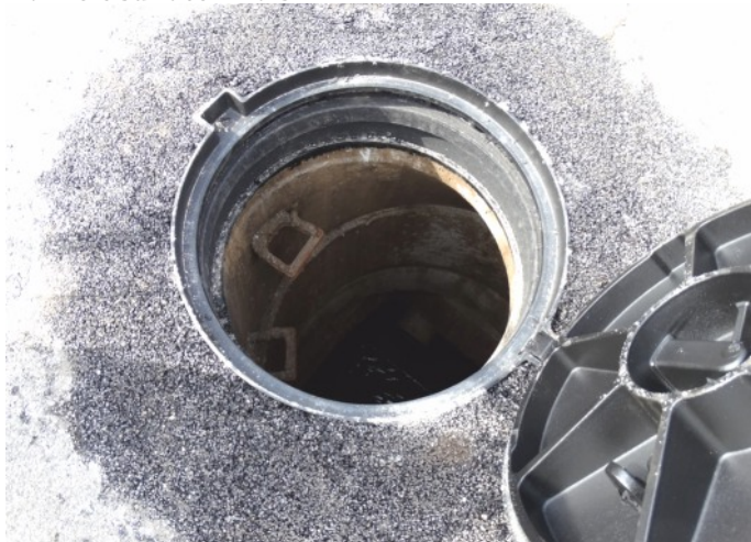
Height adjustment of a manhole done on TVR T System elements
