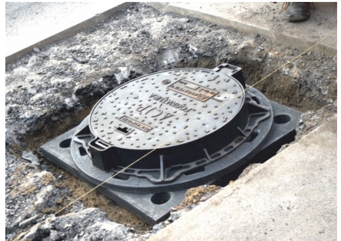
Manhole finial rehabilitation done based on TVR T System adjustment elements
