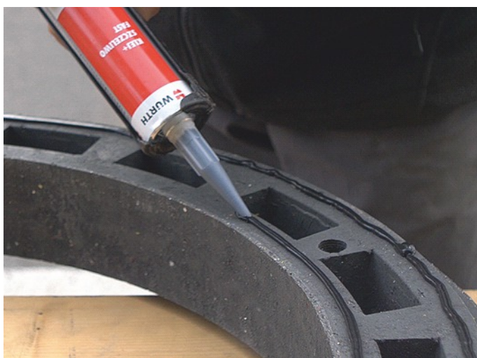
Application of a sealing and binding polymer mass on the surface of lower compensation ring
