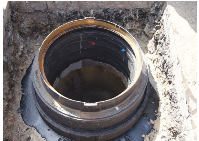
Manhole finial made based on T1R/625 and T1/600 compensation rings along with T1K/600/9/22 wedge rings. Height adjustment 24 cm. Compensation and repair layer made based on poured resin mass.
