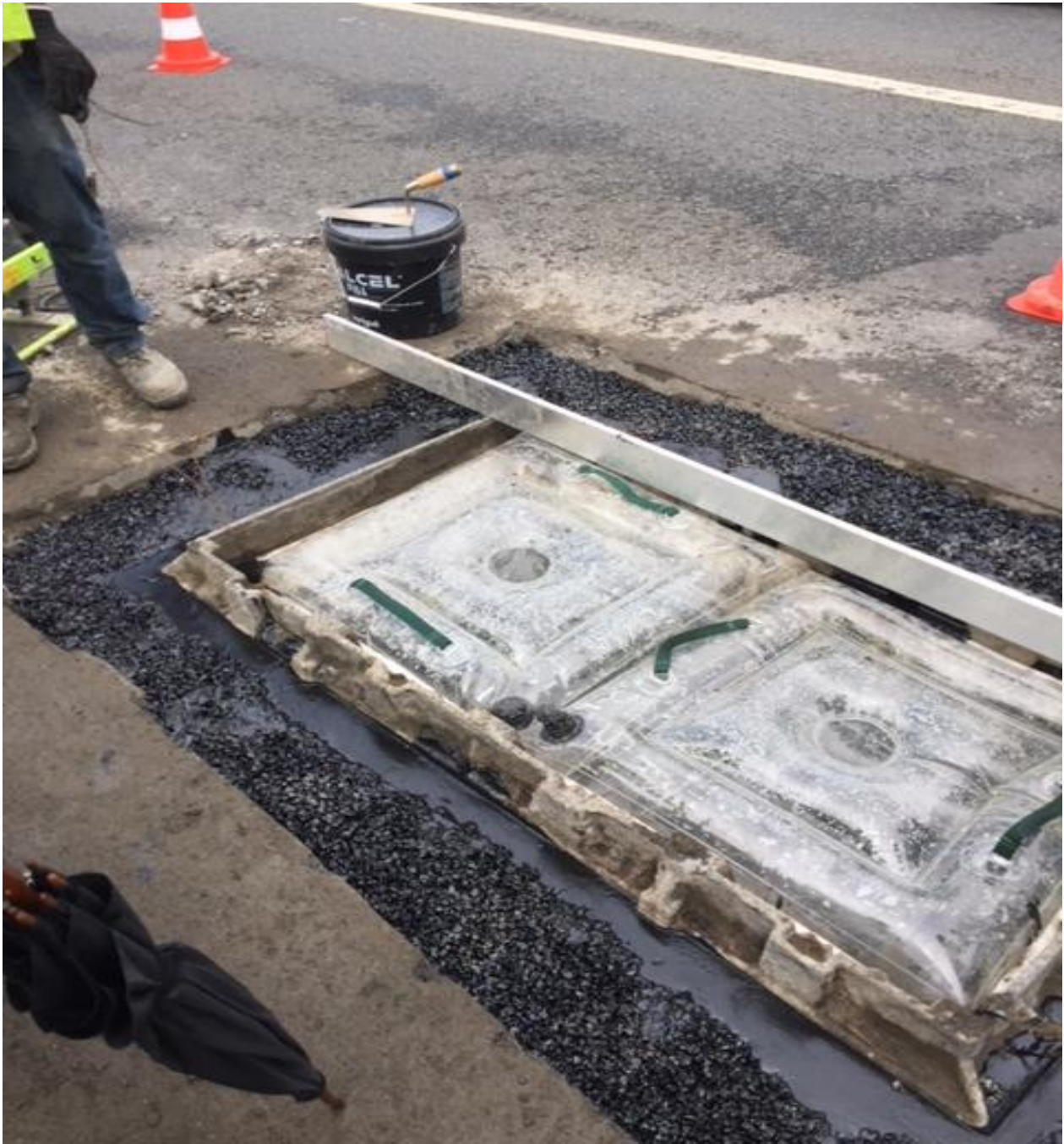
Two pneumatic formwork used to anchor a rectangular manhole on the telecommunication well with the use of polyester resin masses.
