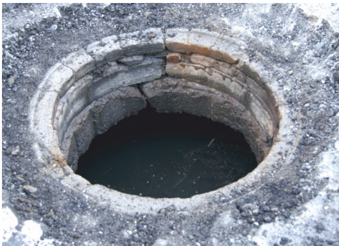
① Intense operation of manhole finial. Complete degradation of compensation rings, concrete levelling and binding mortars, and crack of cover plate. Lack of ability to rehabilitate the finial without the replacement of damaged well cover plate.
