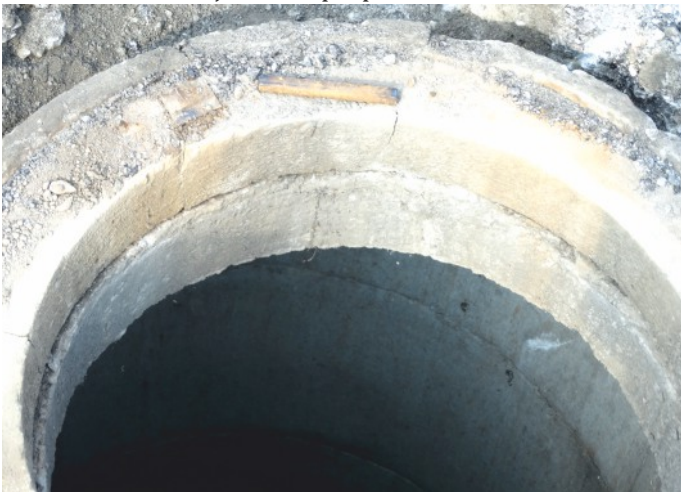
Degradation of structure supporting the manhole. Reinforcement rods as a compensation material - destructive point pressures.
