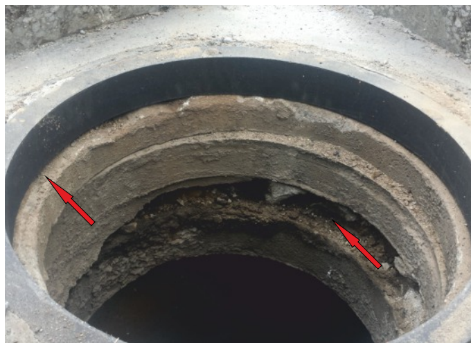
❗ Incorrect ring arrangement (lack of centricity), lack of correct support between the elements
