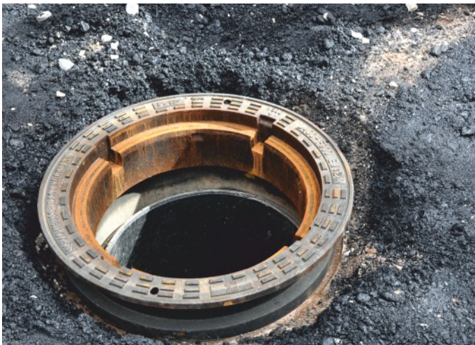
TXS/635/80 adapter/leading ring supporting the EASY LOCK self-levelling manhole during assembly.
