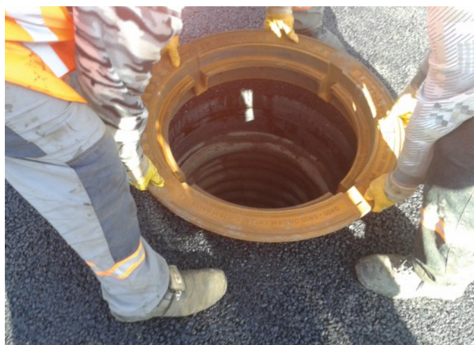
Self-levelling manhole installed in a fortified asphalt surface with the use of TVR T System elements used for construction of Tegra 600 plastic surface well. Jelenia Góra-S-3.
