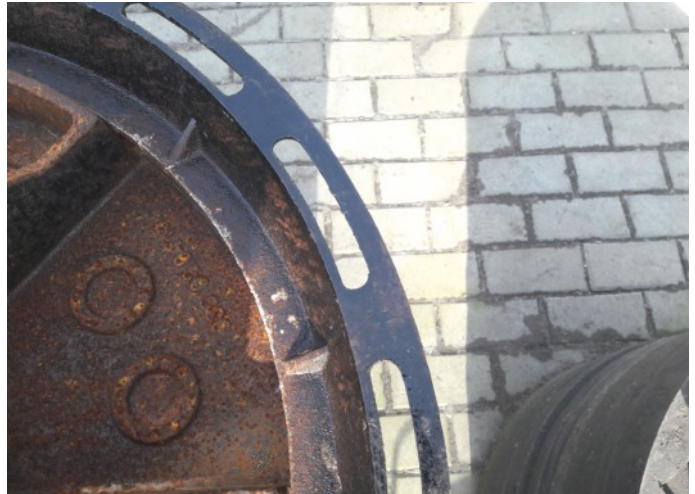
Manhole body with frame plate of load-bearing surface below 1000cm 2 .
