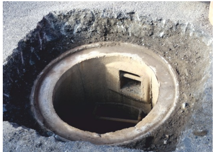
① Choke of DN625 concrete well in a good technical condition that meets the requirements to assemble a surface finial. Small defects and irregularities are to be levelled with levelling layer.
