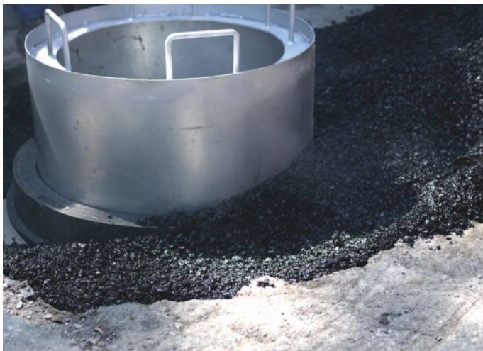
Preparation of a structure supporting self-levelling manhole made from TVR T System elements and hot asphalt mass. The temperature of asphalt mass (170° C) has no influence on the parameters of compensation and leading rings during the installation.
