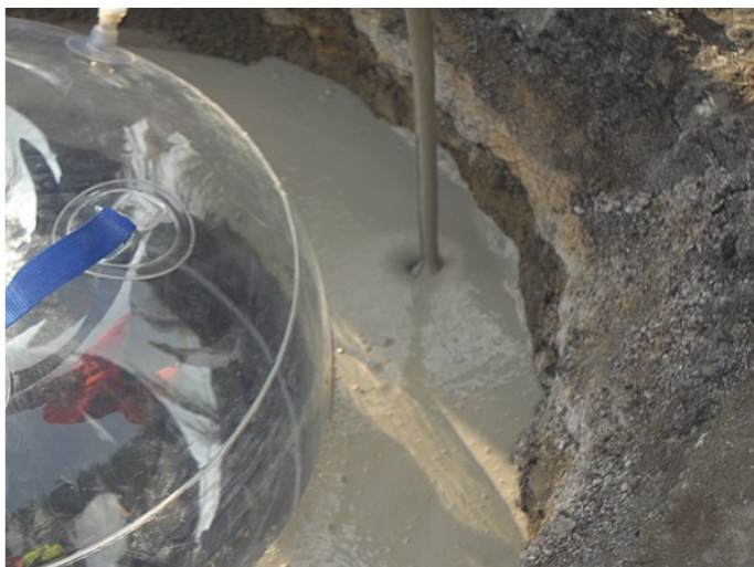
Pu-TS 625 formwork installed in a manhole opening of a well allows to pour the compensation layer.
