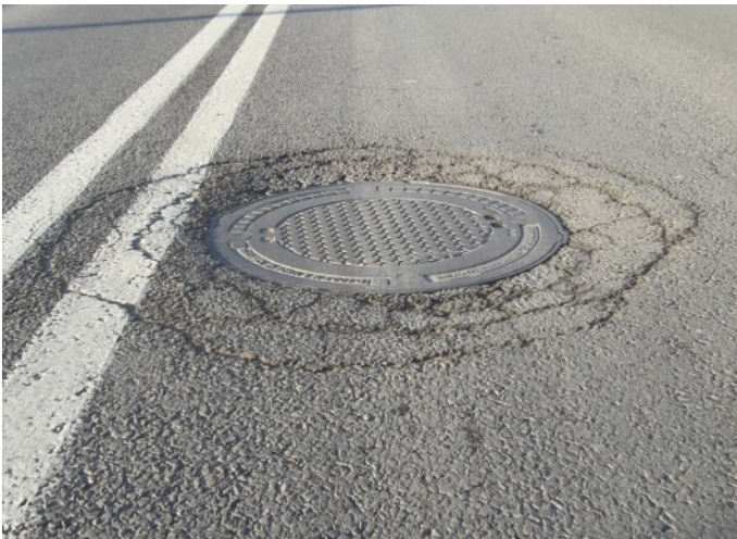
Finial of a sewage well located centrally in the line of vehicle wheel ride. Kr 2-3 traffic load. Elements supporting the manhole are degraded, substructure is damaged, and road surface is cracked.
