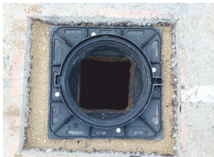
Ductile cast iron manhole with square body plate of 850x850mm set on a T04/850/620/50 foundation slab that provides the full support of the manhole. Manhole anchored to the slab with bolts. Height adjustment is done using T1/600 compensation rings.
