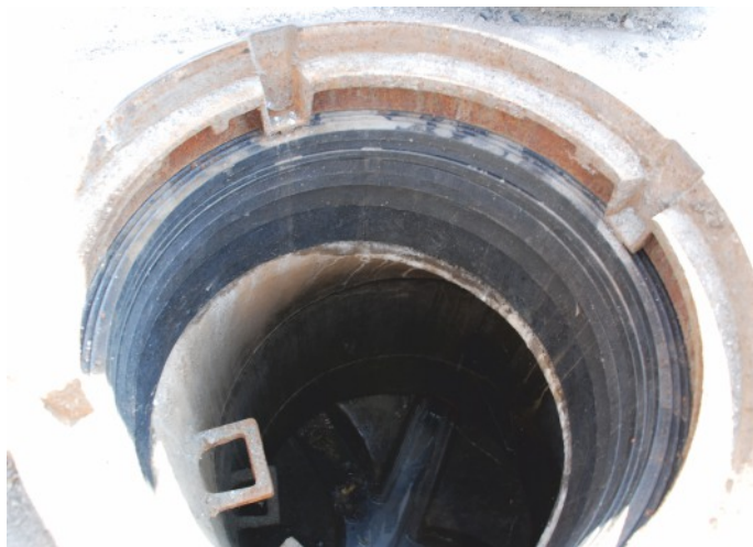
① Structure of a tight surface finial of concrete well with DN625 manhole opening made only on the base of TVR T System plastic rings. Height adjustment of 24,3 cm that refers to surface inclination angle. Lack of joints based on cement mortars. Polymer masses are used as sealing material.
