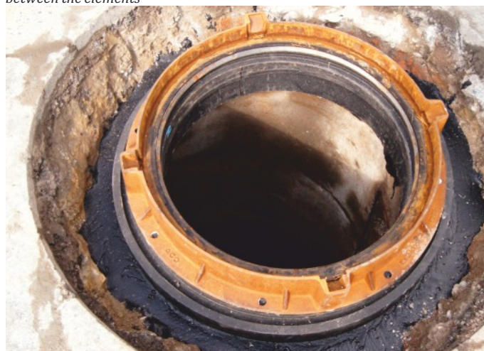
❗ Surface finial of DN600 sewage well with height of 24 cm consisting of mutually compatible T1R/625 and T1/600 compensation rings and T1K/600/9/22 wedge rings.
