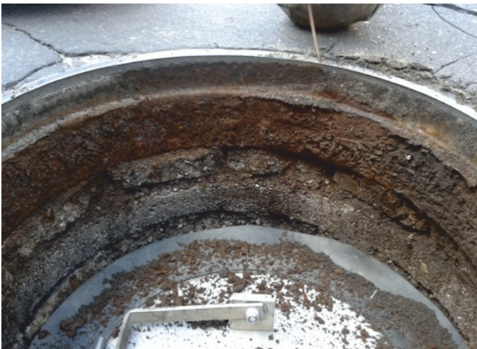
Degradation of a structure supporting a manhole. Concrete mortars in a not bound state and cracked compensation rings. Finial has no tightness and load-bearing capacity.
