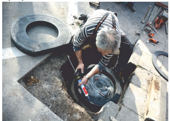
Application of polymer masses between the elements of rehabilitated street drain surface finial.
