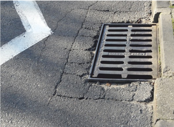
Exploited roadway drain. Location is unfavourable - buses regularly ride over the drain. Surface cracks are caused by the lack of finial tightness and lack of substructure.
