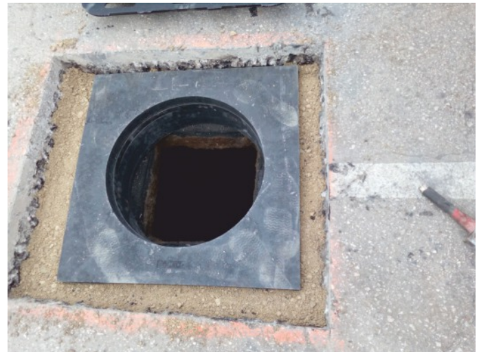
T04/850/620/50 foundation slab installed on T1/600 compensation rings and surface substructure, prepared for assembly of a manhole with 850x850 square plate.
