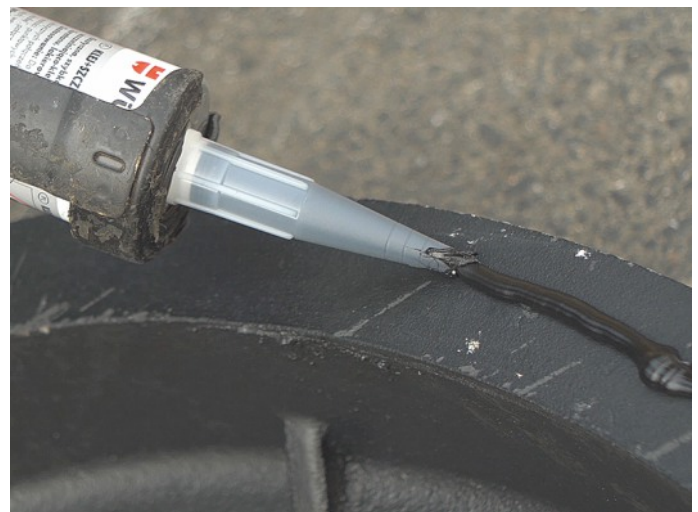
Application of a sealing and binding polymer mass on the surface of lower load-bearing plate of a sewage manhole
