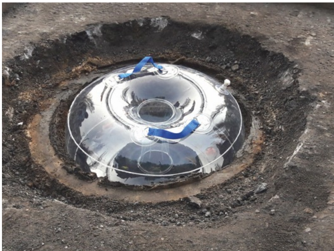
Before commencing the disassembly works of a finial, the pneumatic formwork can be used as a protection against contamination.
