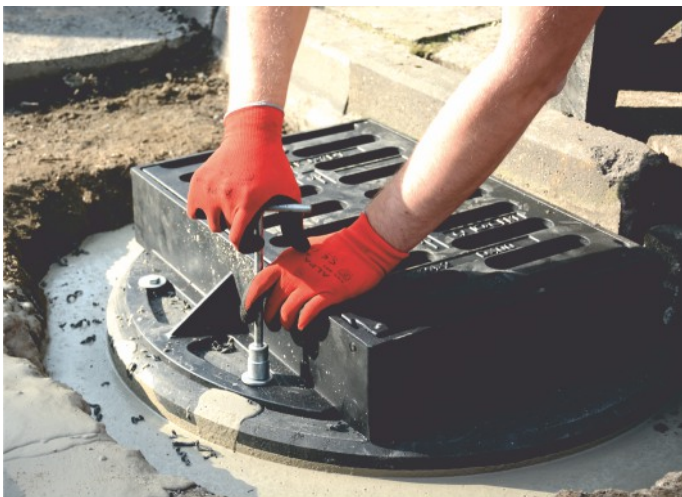
400x600 street drain, flange 3/4, installed on a TX/765/410/80 adapter. Drain anchored to the adapter. Adapter is secured with poured mass poured around the repaired finial. Poured mass constitutes as a substructure for road surface.
