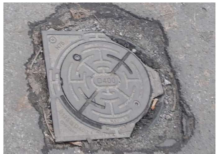
⚠ Telescope manhole for DN315 well damaged due to the lack of even and permanent support.
