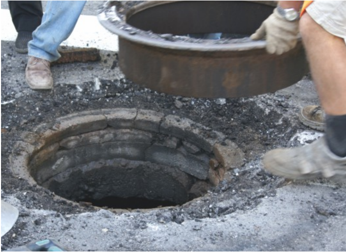
Disassembly of a self-levelling manhole with smaller frame support surface (about 1600cm 2 ) installed directly on concrete elements! Negative weather conditions. Operation period 1.5 year
