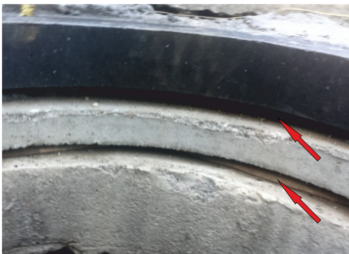
❗ Unacceptable lack of support for compensation rings, adapters. Finial does not provide load-bearing capacity, tightness, and safety of the structure!
