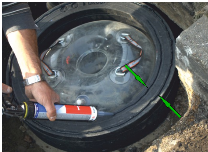
❗ Application of flexible sealing and binding polymer mass between all the adjustment elements and cast-iron.
