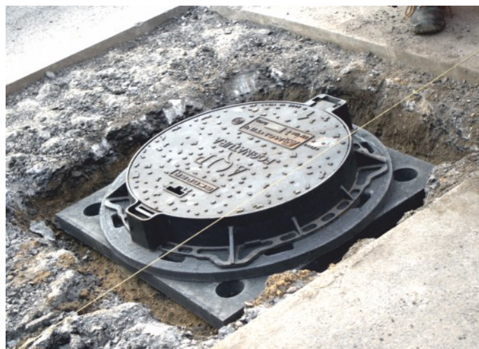
Manhole finial rehabilitation done based on TVR T System adjustment elements
