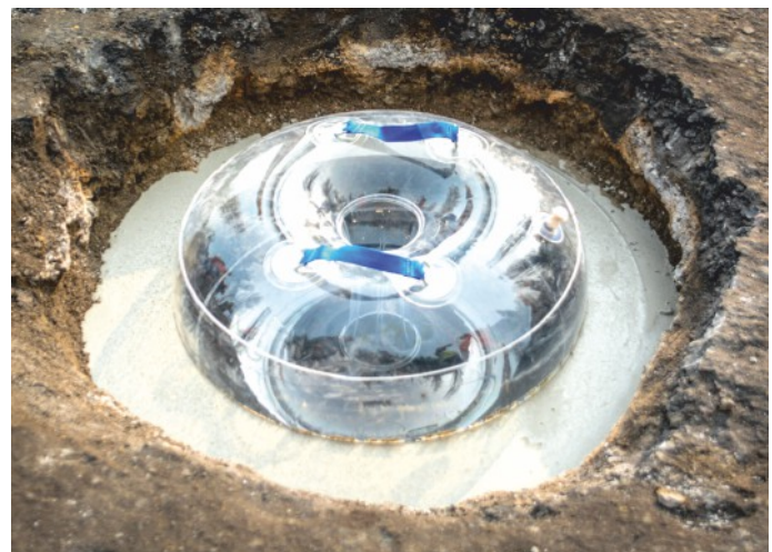
① Application of a cement-based, fast-setting, flexible repair and levelling mass. Exceptionally short binding time allows to immediately assemble the surface finial elements.
