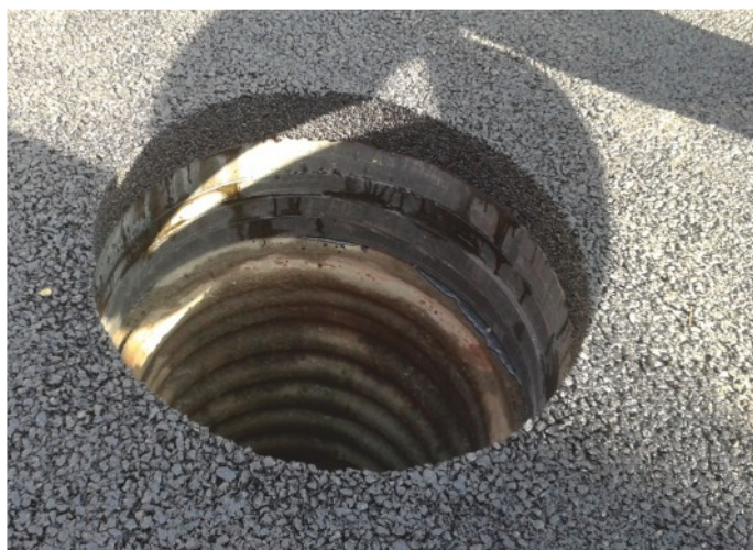
Surface finial of Tegra 600 well made from TVR T System elements (T1/700/50 compensation rings and TXS/700/80 leading ring) prepared for the installation of self-levelling manhole. Jelenia Góra-S-3.
