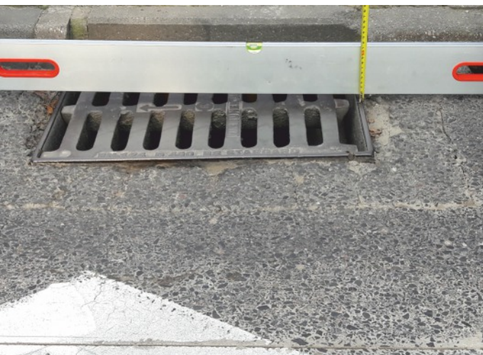
Verification of technical condition of a drain. Drain is collapsed. The grate in the frame is lowered.
